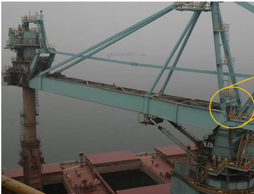
Boom B.C Motor
